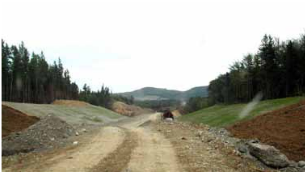
Areas stabilized as work progresses - Good Work Progression
