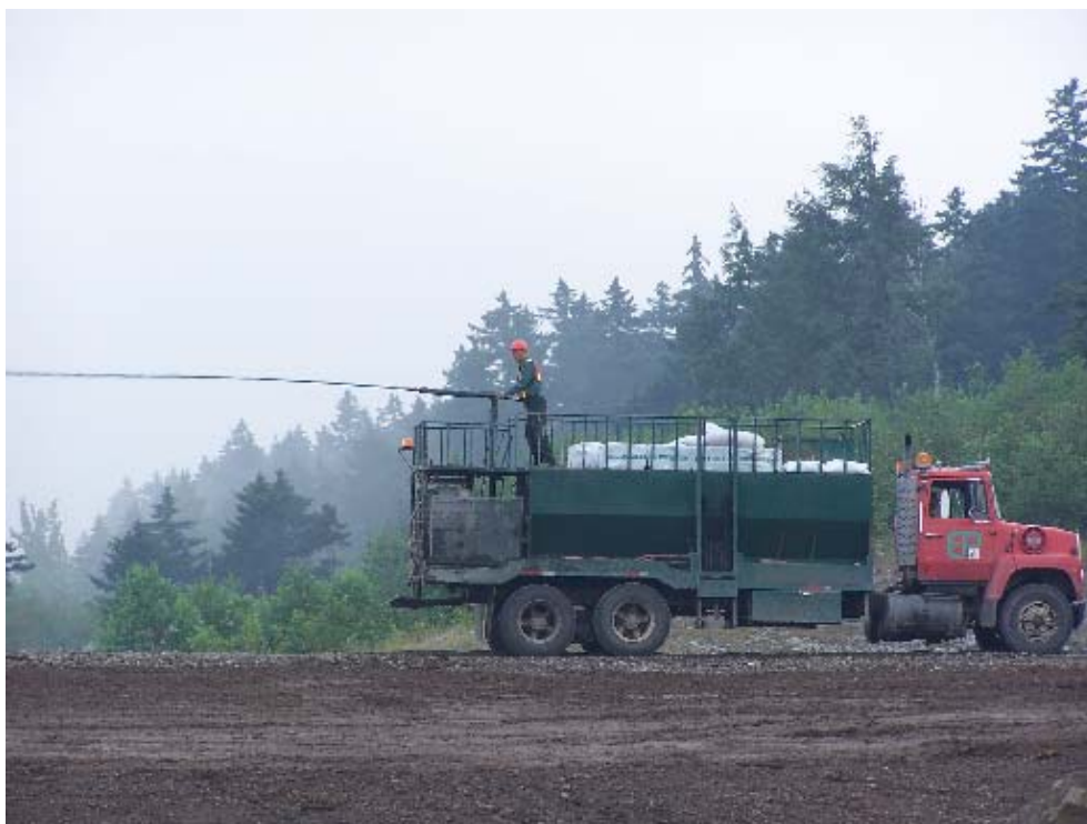
Hydroseeding – Application by mechanical means
