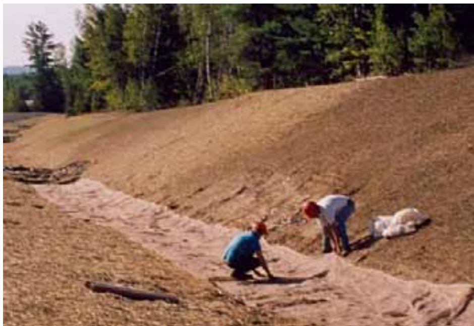
Jute mat installation in ditch.
