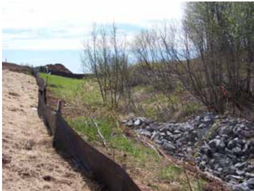
Proper installation of sediment control fence at toe of fill.
