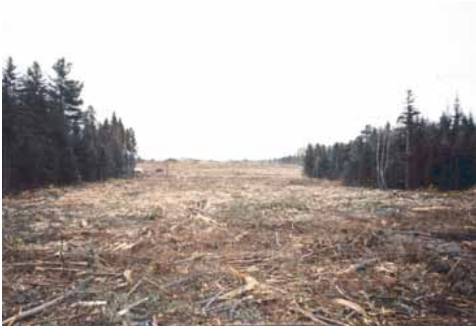
Properly cleared area. Note that there are no standing trees
