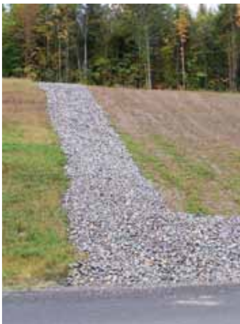
Completed Flume (Slope Drain)
