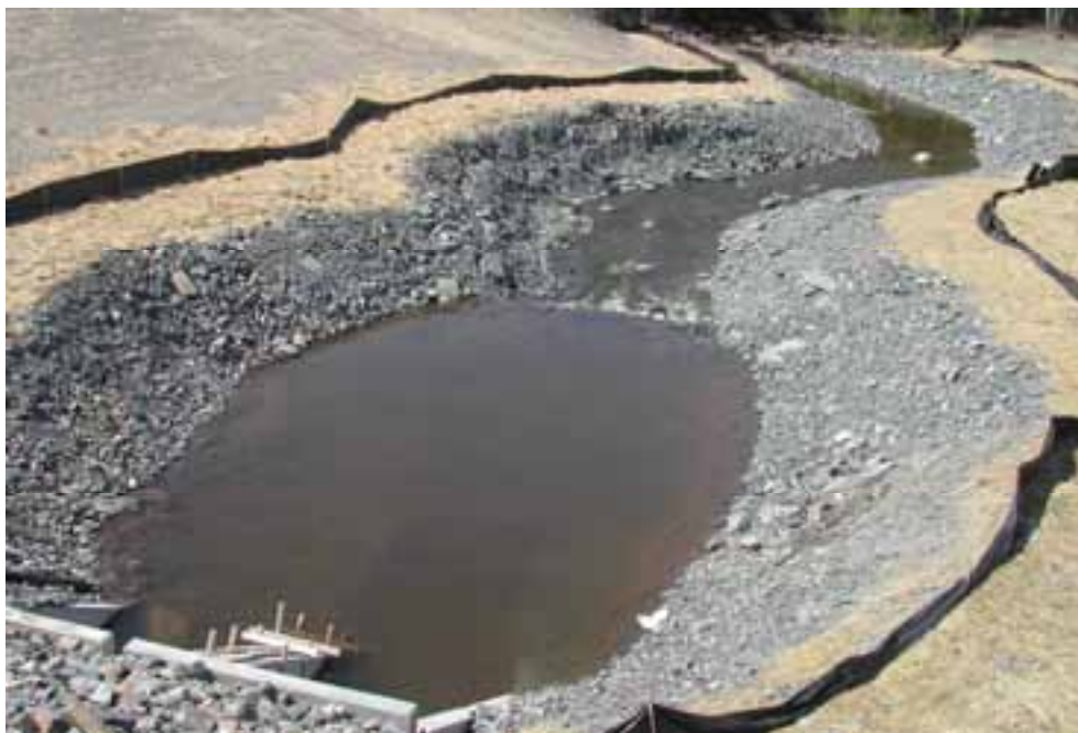
Energy Dissipator Pool
