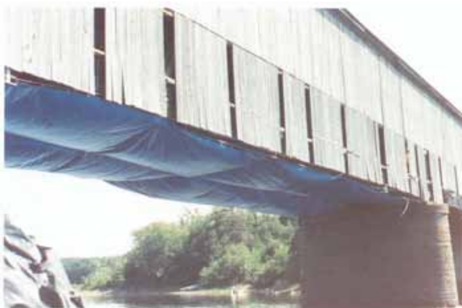
A properly protected watercourse during chipsealing operations.
