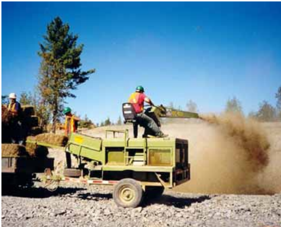
Mulching – Application by mechanical means.
