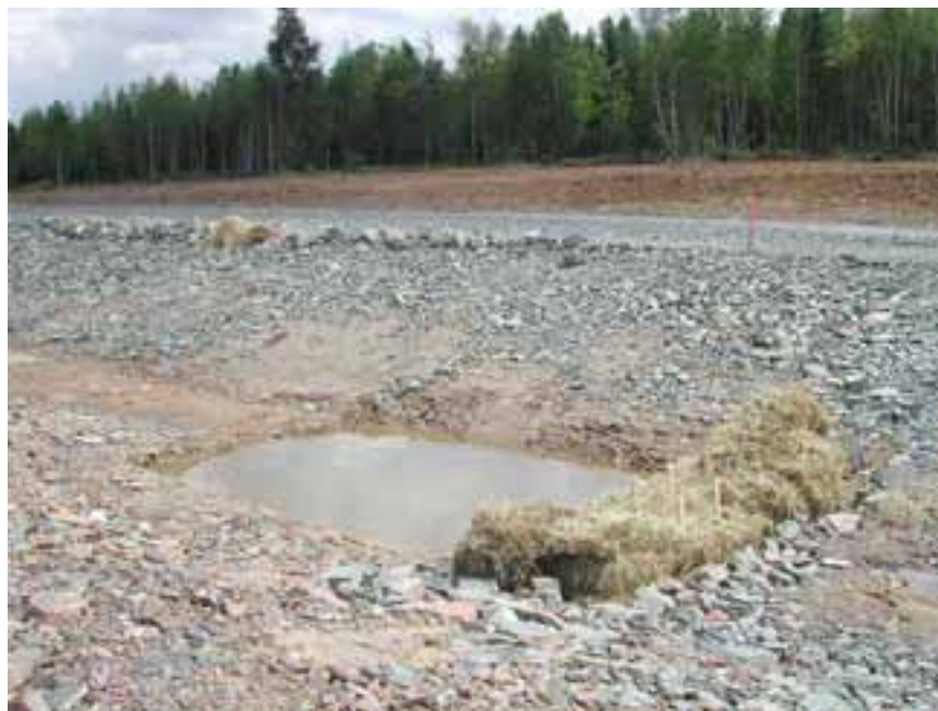
Completed Type D Erosion Control Structure
