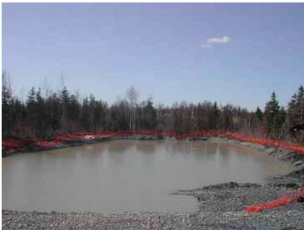
Large Sediment Pond with Safety Fence
