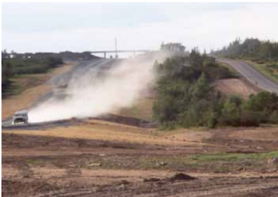
Worksite that requires dust suppressants.
