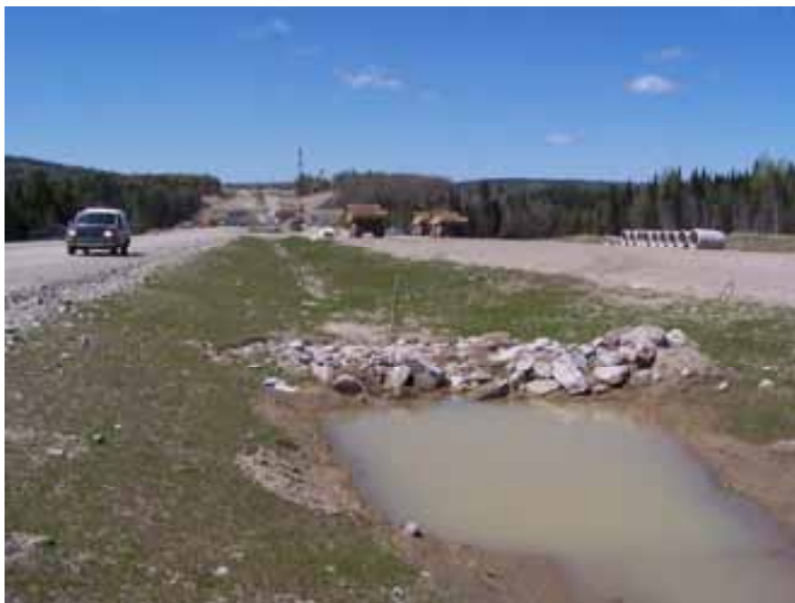
Completed Type B Erosion Control Structure
