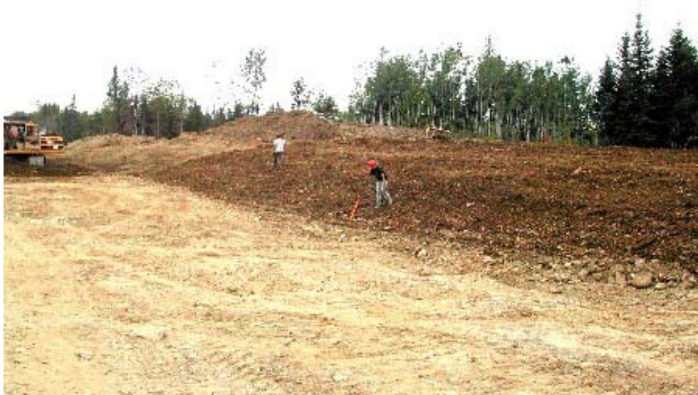
Topsoil on backslope. Roots being removed by hand.
