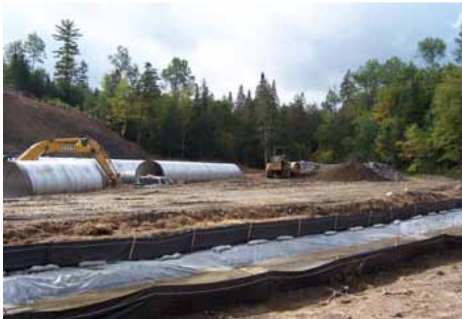
A temporary plastic-lined diversion channel.
