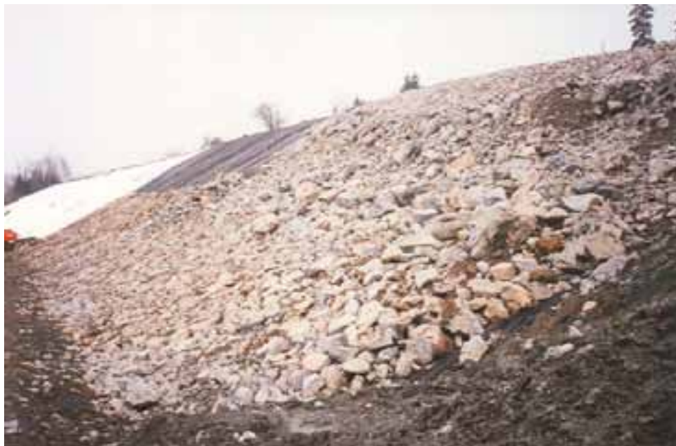
Placement of riprap on backslope.
