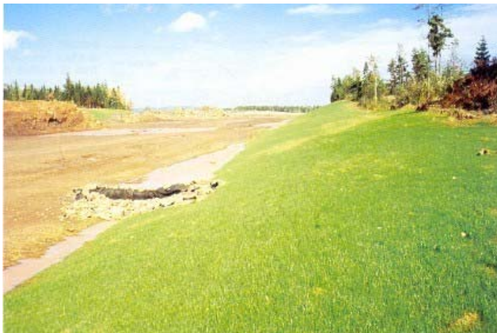
Completed Erosion Control Structure C
