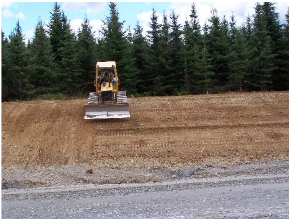
Back-dragging topsoil.
