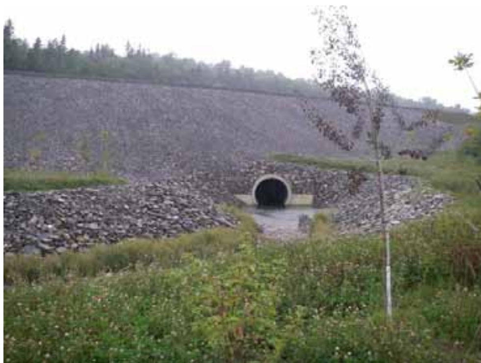
Permanent Stabilization of Worksite, including fill foreslope erosion protection
