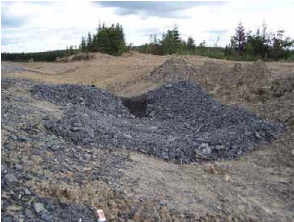
Completed Type A Erosion Control Structure
