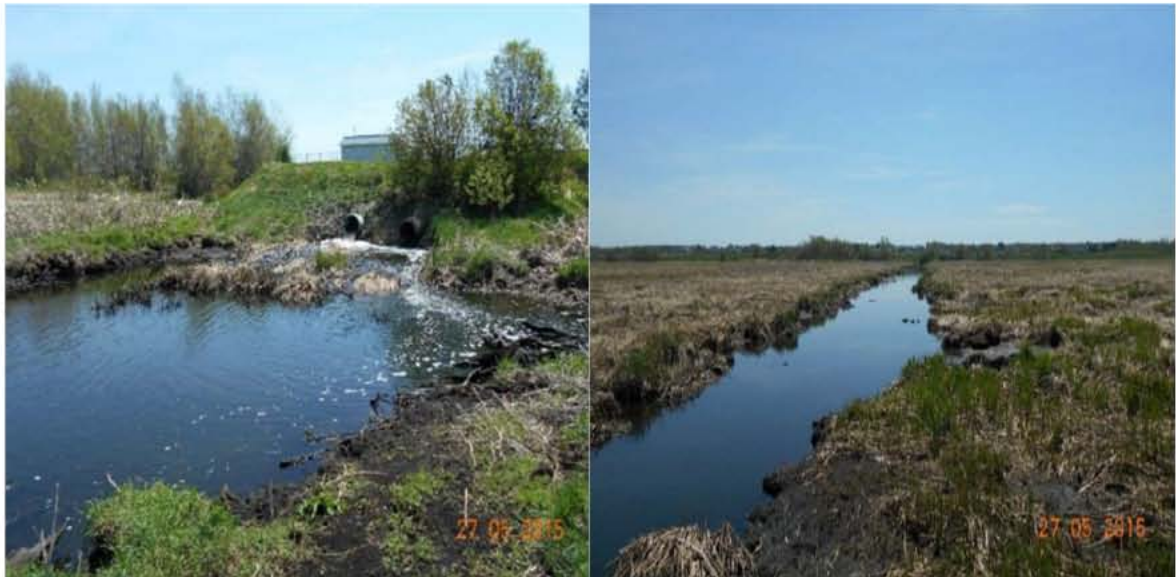
Figure 2 – Existing Discharge and Outfall Trench
