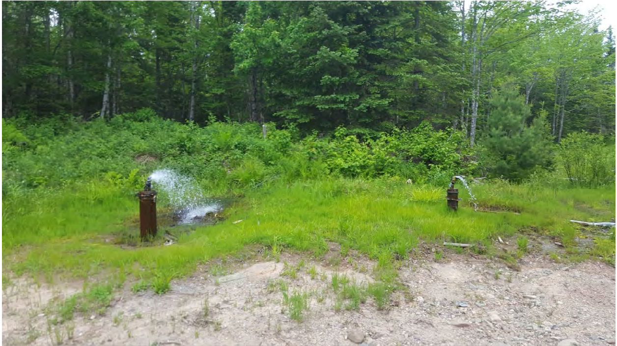
Photo 1. Test wells located along access road and adjacent to the west central portion of Wetland 1.
