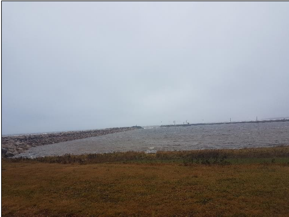
Photo 6. Looking north at breakwater.
