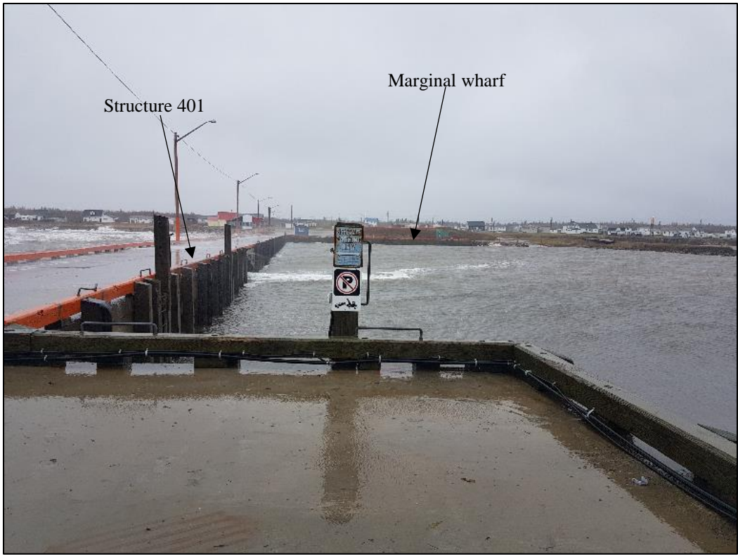
Photo 9. Looking south at wharf structure 401 and the marginal wharf.
