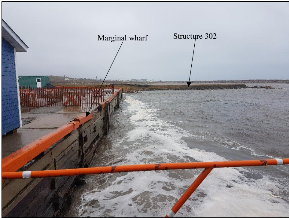
Photo 7. Looking west at structure 302 and marginal wharf.
