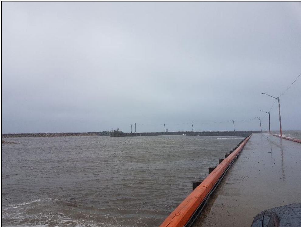
Photo 8. Looking north from wharf structure 401 (inside basin).
