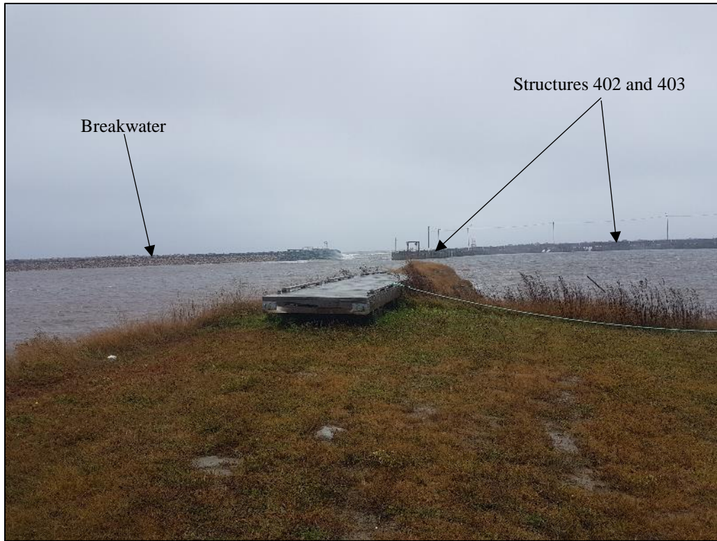
Photo 3. Looking north at the wharf structures 402 and 403 and breakwater.
