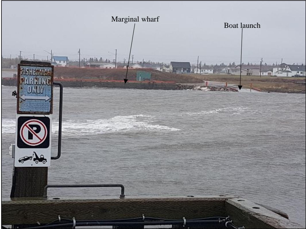
Photo 10. Looking south at marginal wharf (structure 404) and boat launch (structure 502).
