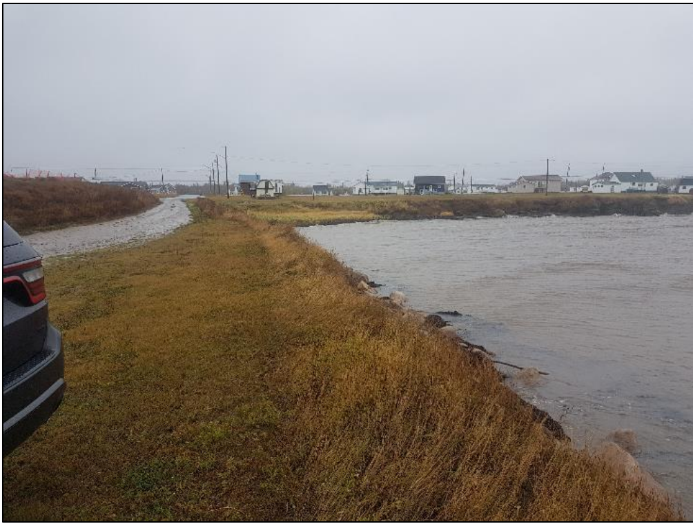
Photo 5. Looking south from structure 302.
