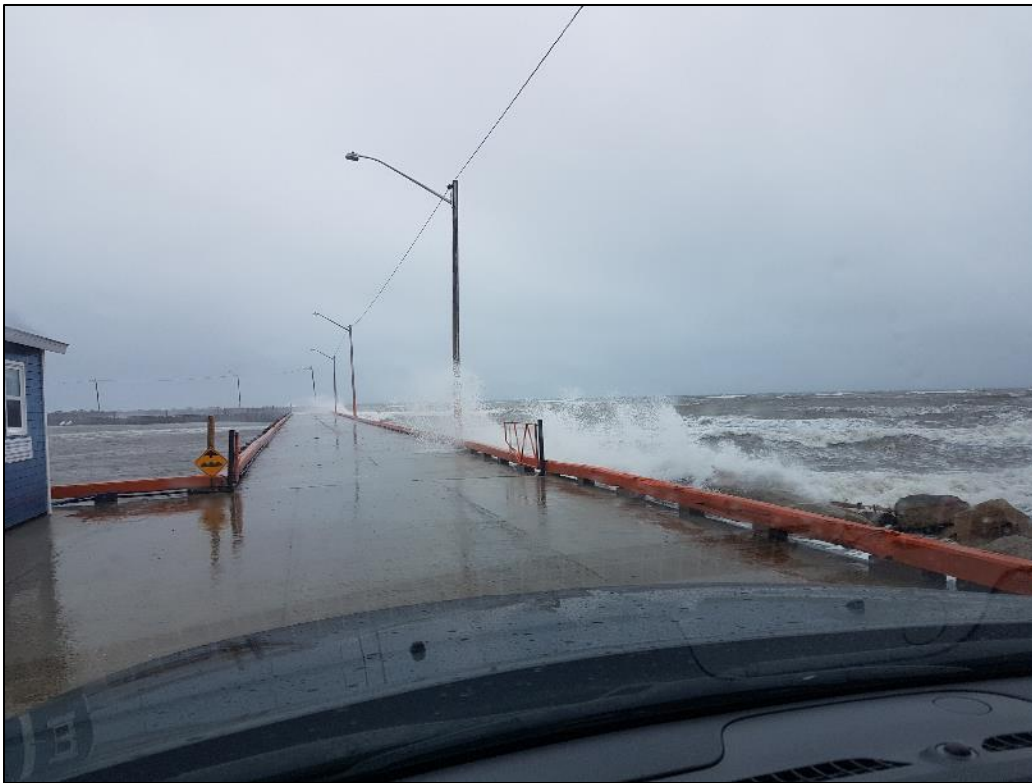
Photo 1. Structure 401 looking north.
