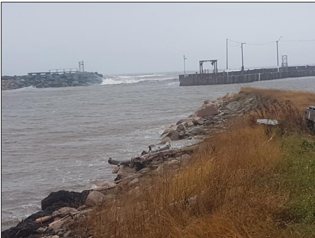
Photo 4. Looking north at breakwater and harbour channel.
