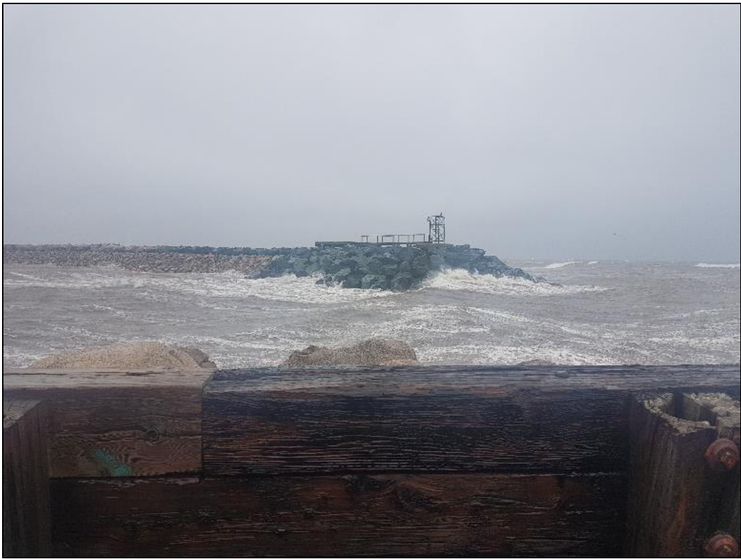
Photo 11. Looking west, from wharf 403, at the breakwater.
