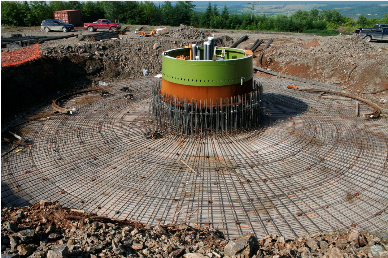
Figure 2-3: Construction of a concrete foundation at Natural Forces' Fairmont Wind Farm.
