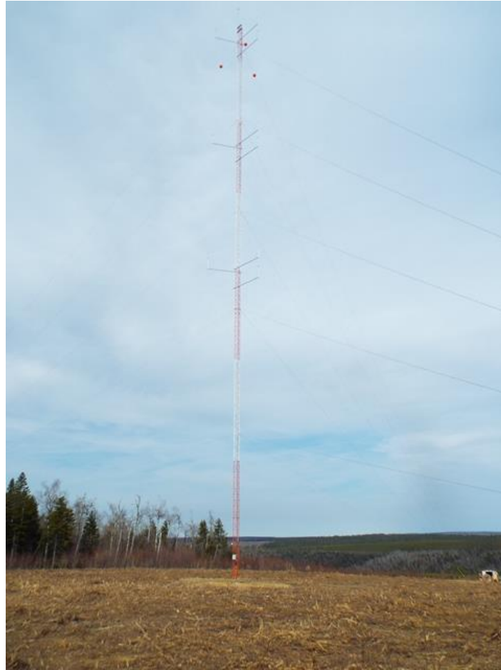
Figure 4-3: The 80m Met Tower installed in April 2017
