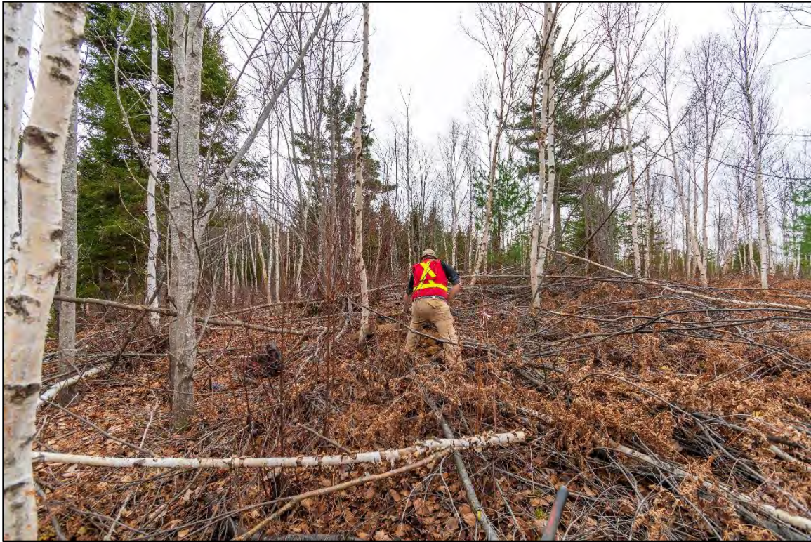
Figure 26: Updated area at Structure 12.
