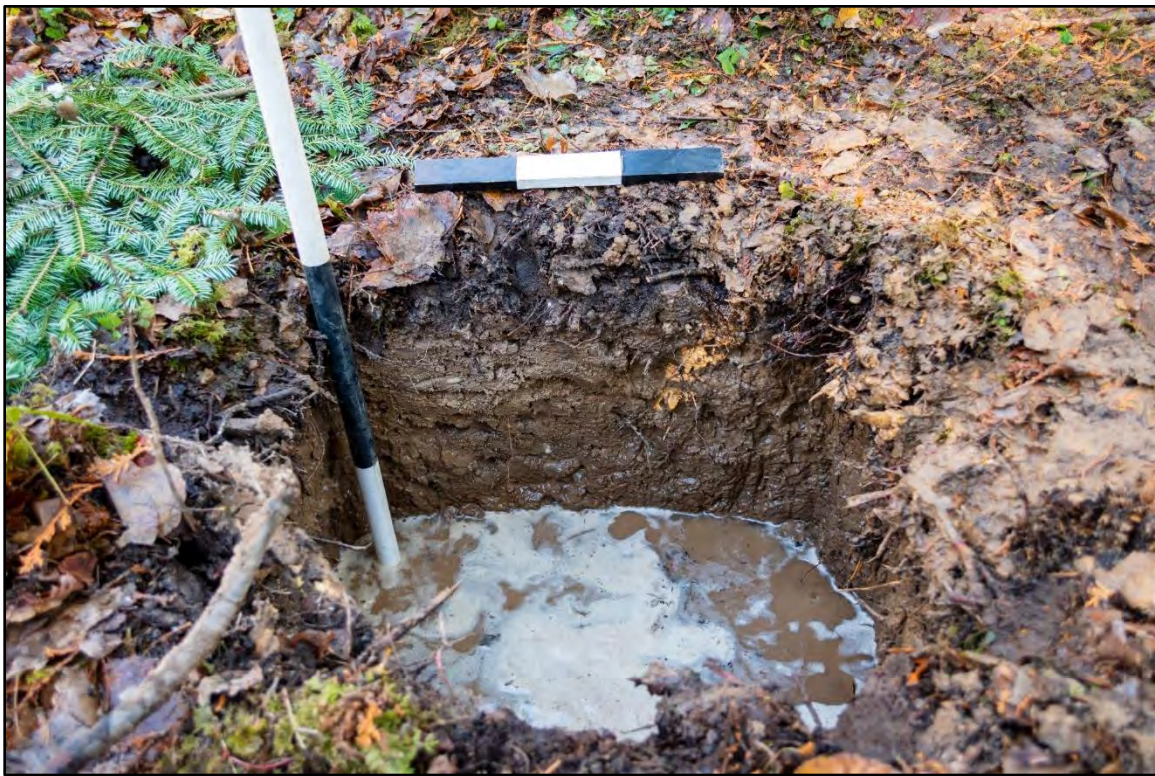
Figure 10: Test pit on east side of poles trench at Structure 15.
