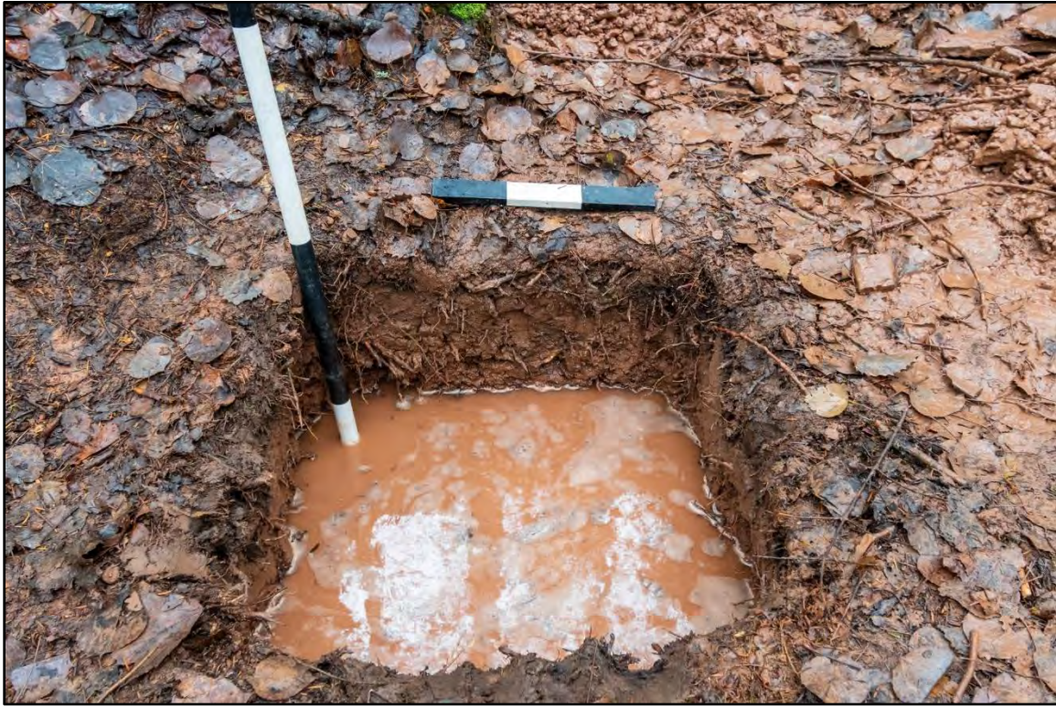
Figure 12: Test pit on east side of poles trench at Structure 16.
