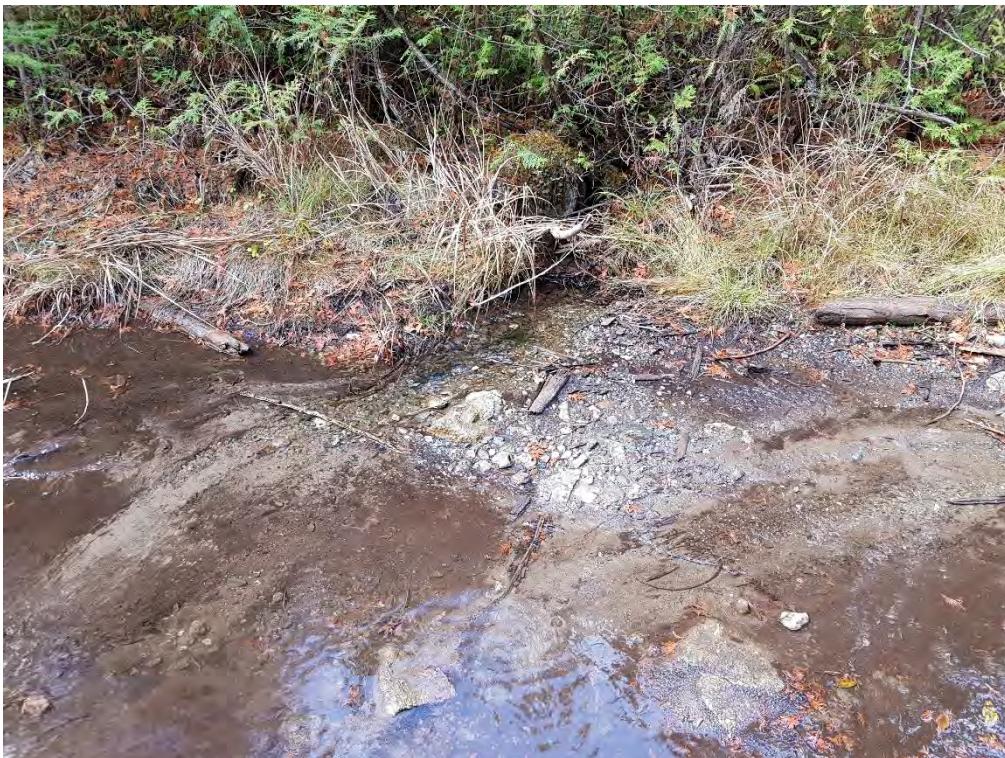
Photo 20. WC1 has deposited coarse material into the ATV trail, during high volume run-off events. Photo facing upslope, where the sub-channel enters the trail.
