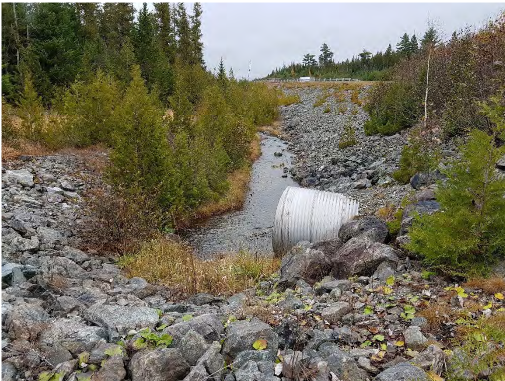
Photo 24. Parts of WC4 near the highway have been reconstructed.
