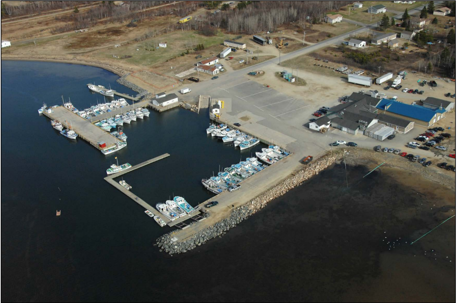
Figure 2: Oblique aerial photo of Val-Comeau DFO-SCH, Gloucester County, New Brunswick
