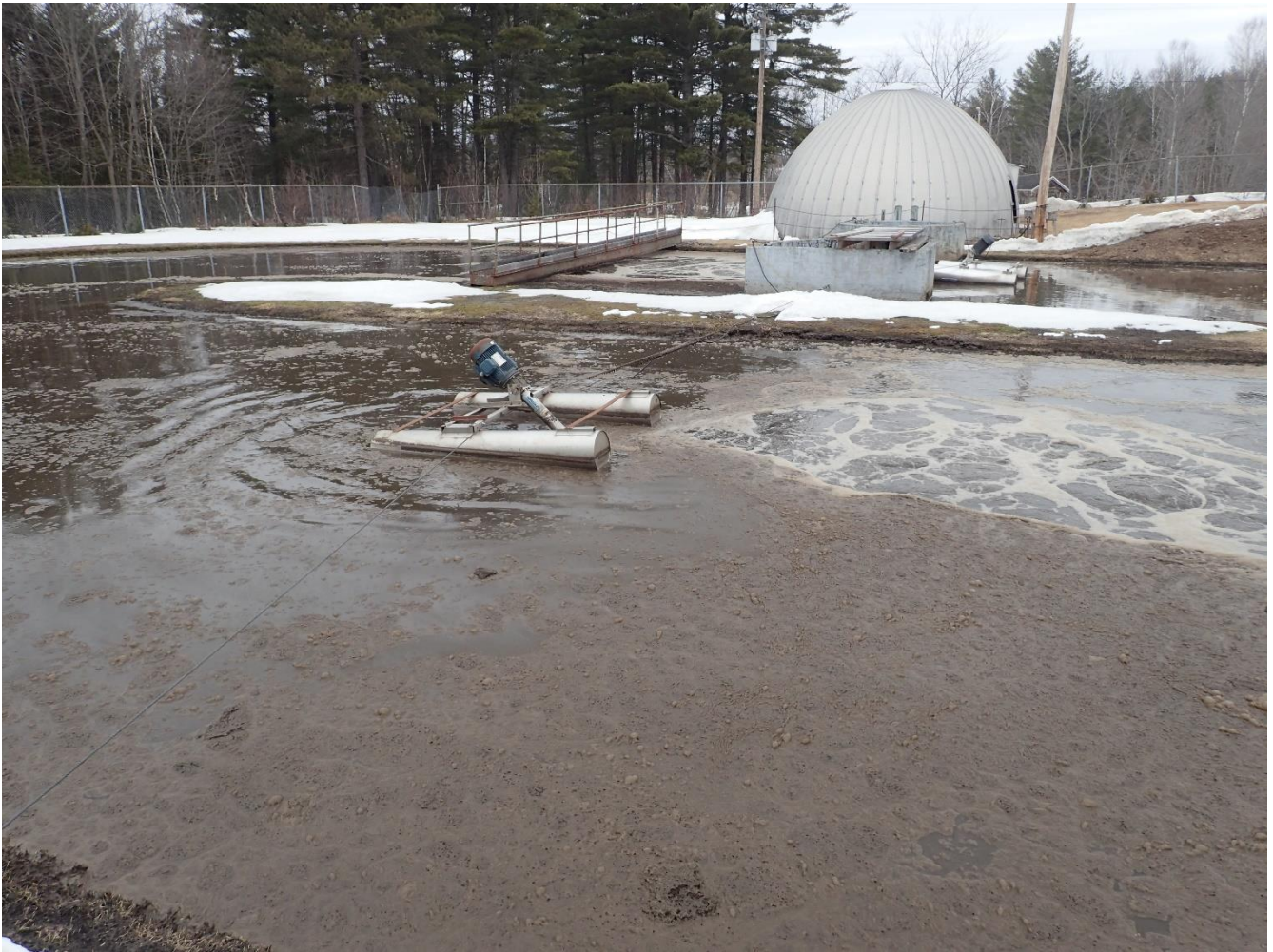
Figure 11 - Looking north from the oxidation ditch
