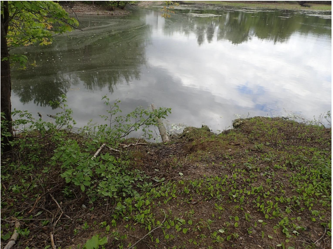
Figure 14 - Looking down the current outfall alignment
