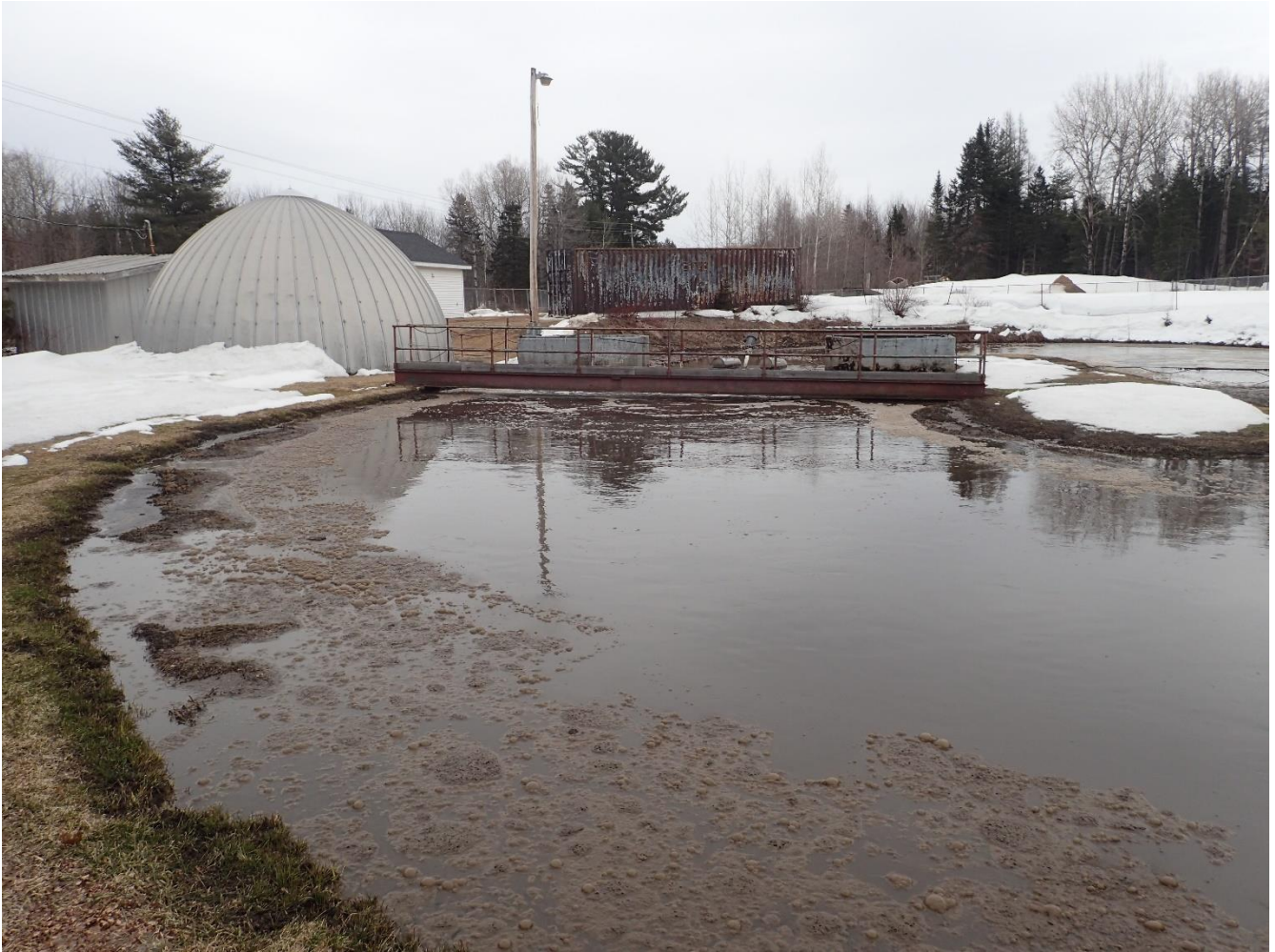
Figure 10 - Current WwTF from western edge end of ditch
