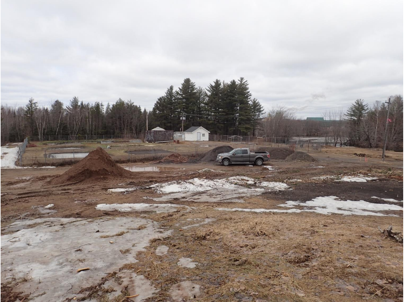
Figure 9 - Photo of Existing WwTF
