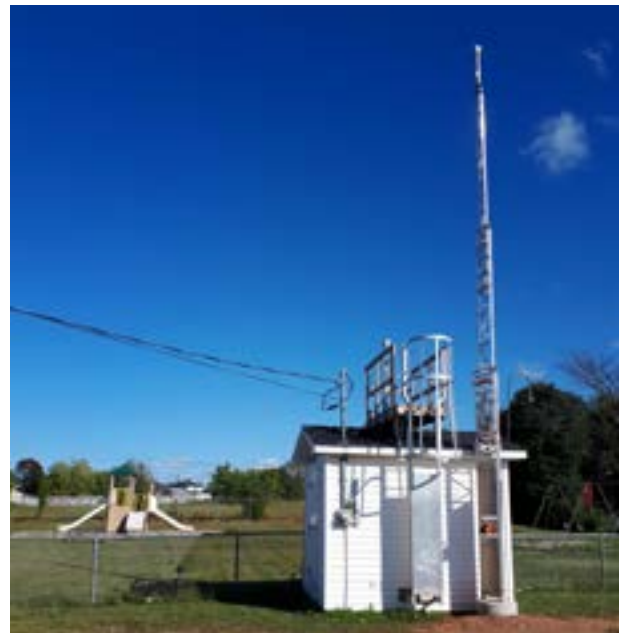
Air Quality Monitoring Station (Bathurst)
