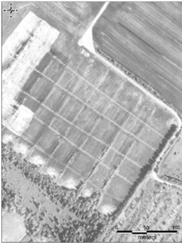
Figure 10. Aerial photo of Chemin-du-Lac restoration site, Québec. To achieve good distribution of water over the site, chessboard berms were created because of the complex slopes and short fields, forming cells about 30 m across. (Photo: Premier Horticulture Ltd.)
