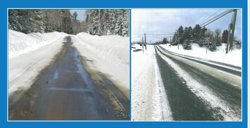
Objective: Bare center strip or bare wheel path within 48 hours after end of storm
