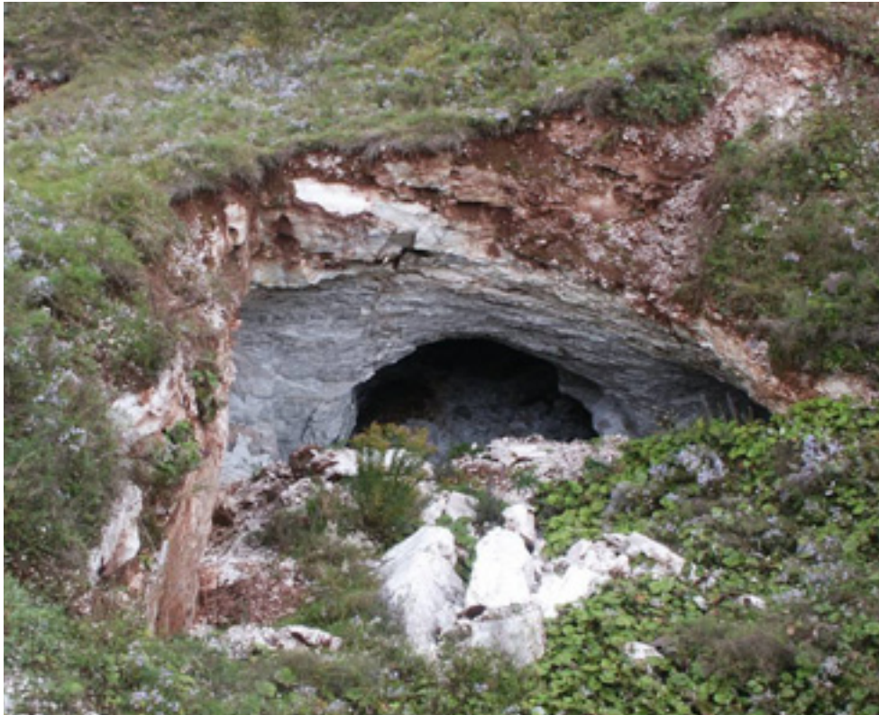
Figure 22. Partial crown collapse, exposing supportive pillars over former underground gypsum workings near Hillsborough, Albert County, southeastern New Brunswick
