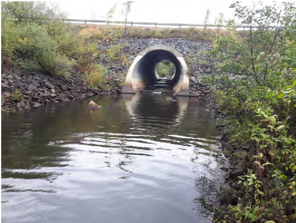
Photo 15: View of Oxford Brook under Saint Agnes Street, facing north (September 28, 2017).
