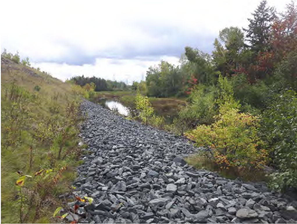
Photo 16: View of eastern bank of Oxford Brook, facing south (September 28, 2017).
