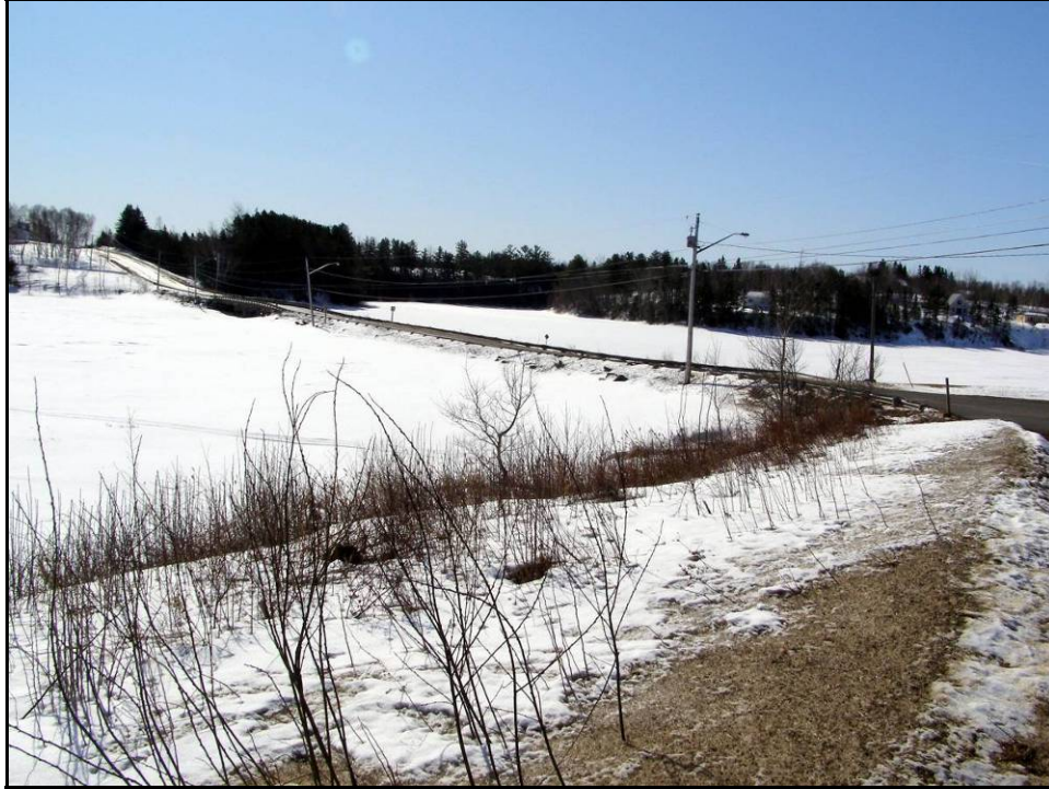
Figure 3a. Looking south/southwest, Little Tracadie River bridge with longest portion of causeway in mid-foreground. Trout Stream enters the Little Tracadie River just to the right (west) of south bank causeway landing. Immediate foreground illustrates the extent of the fill deposit banking the east side of the Thomas curve (March 2012).
