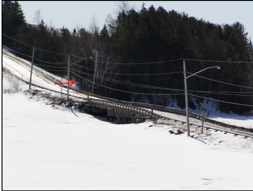
Figure 13a. Looking southwest at south end of causeway. Red arrow points to edge of gravel pit. (March 2012)
