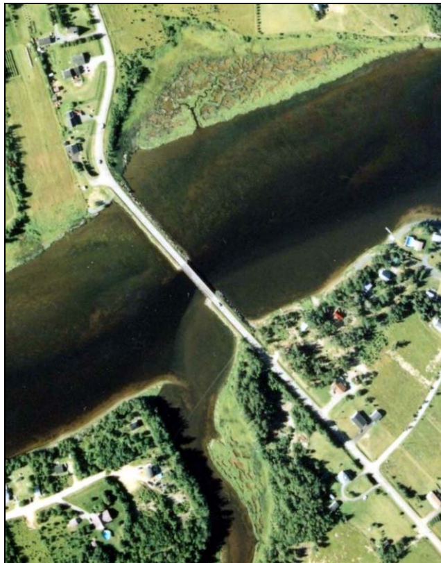
Figure 3b: Little Tracadie River bridge (2002 Aerial DNR 512-118) North at top of photo. Trout Stream enters the Little Tracadie River just west of the southern end of the causeway.
