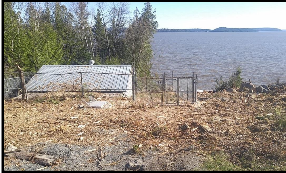
Photo 1: Looking north towards existing WWTF building from access/parking area.
