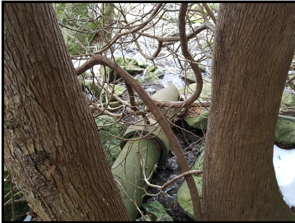
Photo 2: Existing concrete effluent pipe, looking at outfall location on bank of Saint John River. Photo taken prior to clearing activities.
