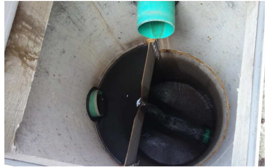
Weir in outlet manhole
