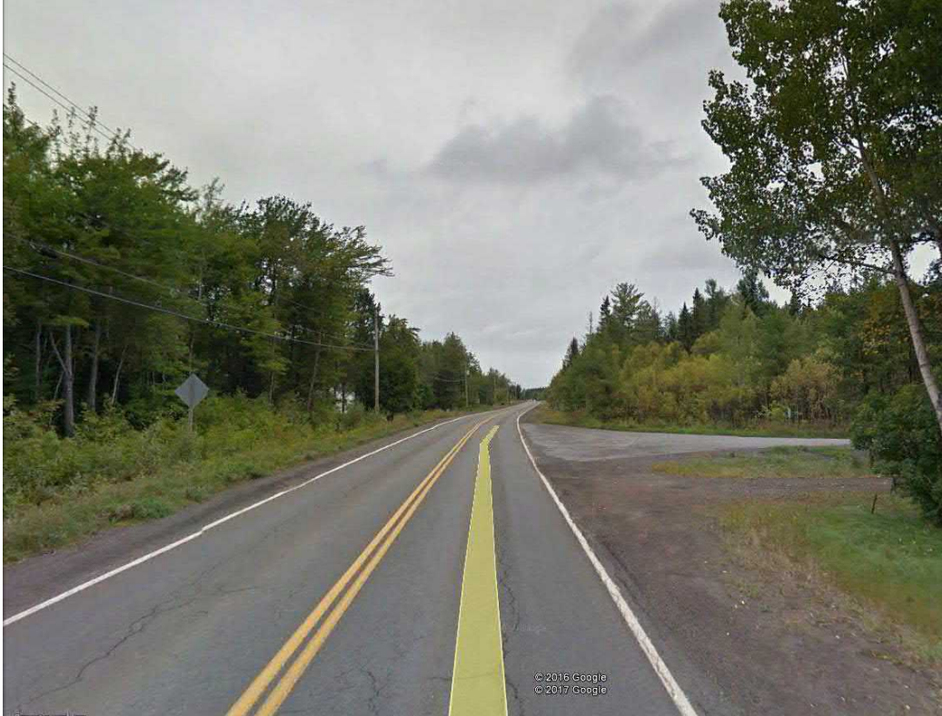
Photo no. 8: Route 10 at entrance to site access road (Google Earth).
