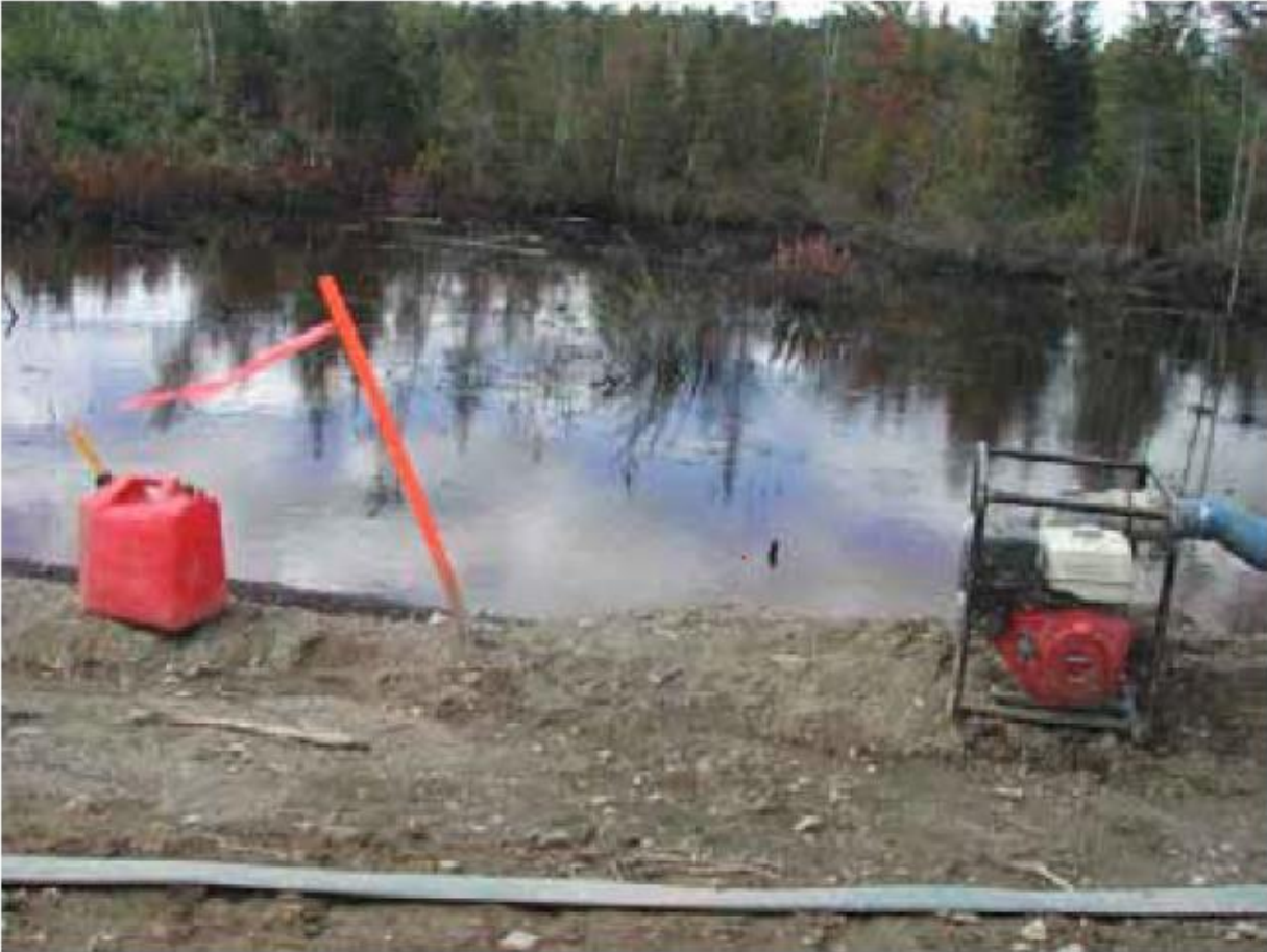
Petroleum products stored too close to a watercourse.
