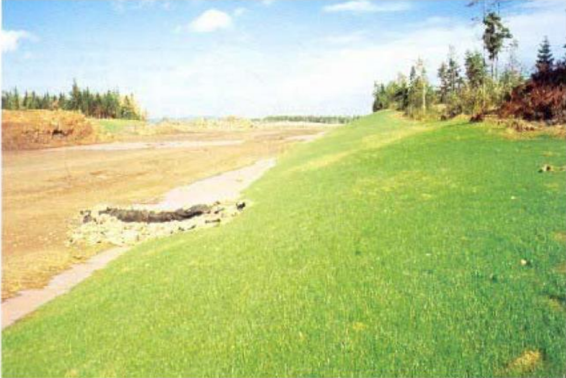
Completed Erosion Control Structure C
