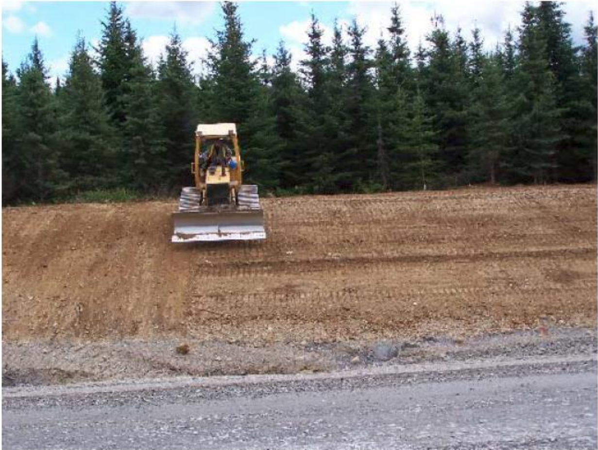
Back-dragging topsoil.
