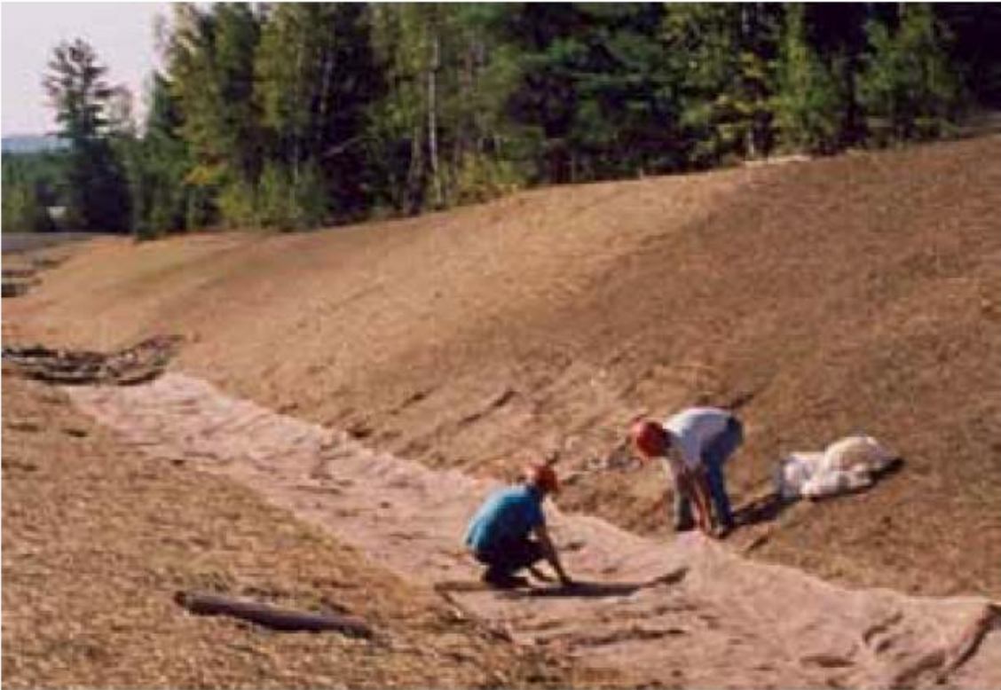
Jute mat installation in ditch.
