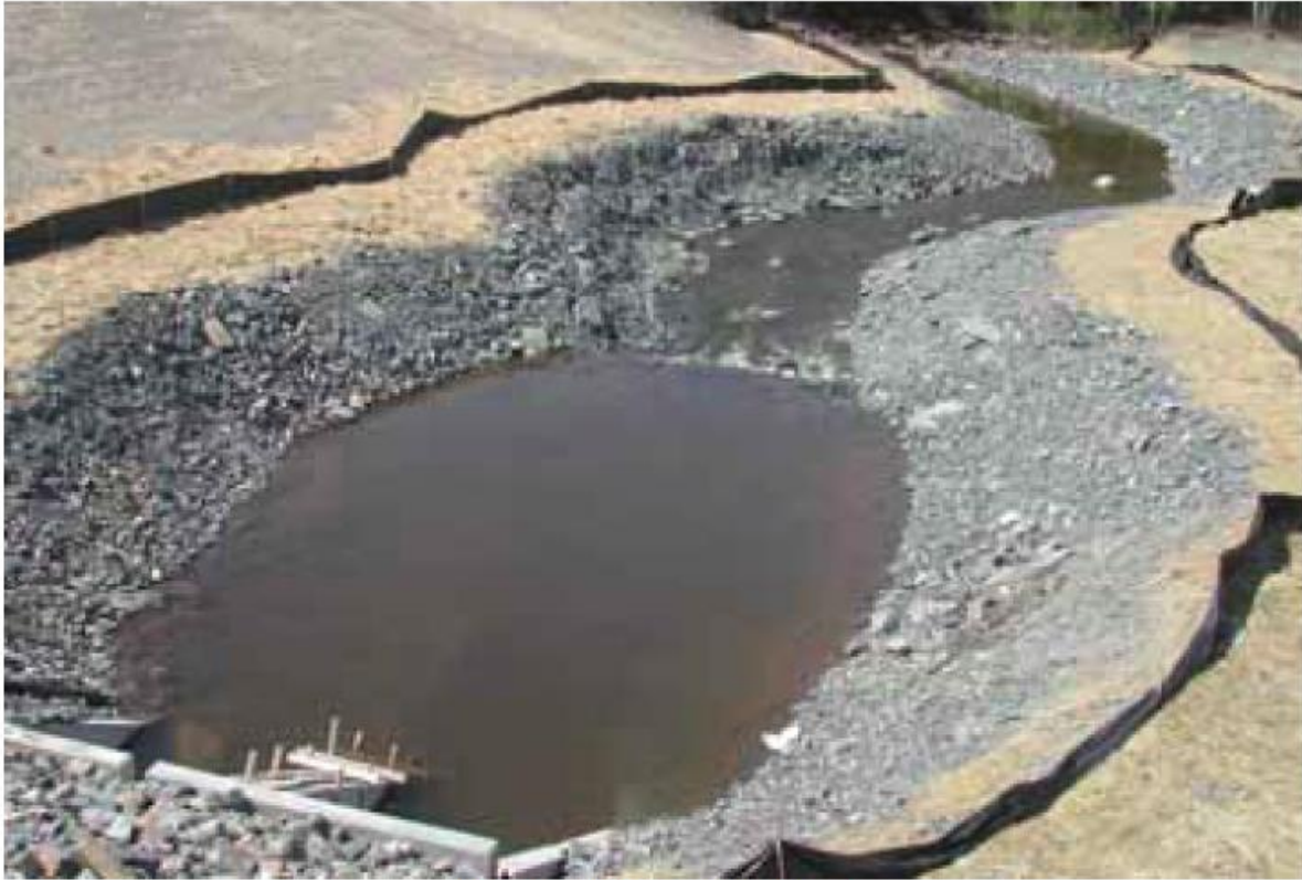
Energy Dissipator Pool
