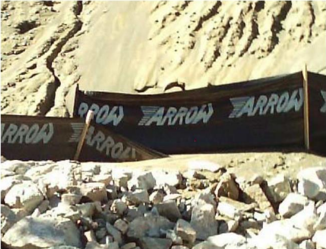
Sediment passing around end of fence.
