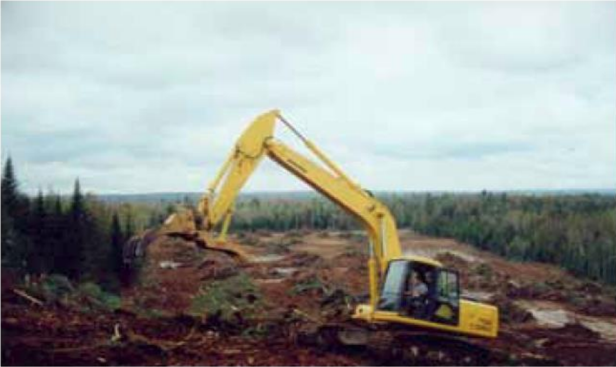
Root rake attached to excavator used to remove roots and stumps only.
