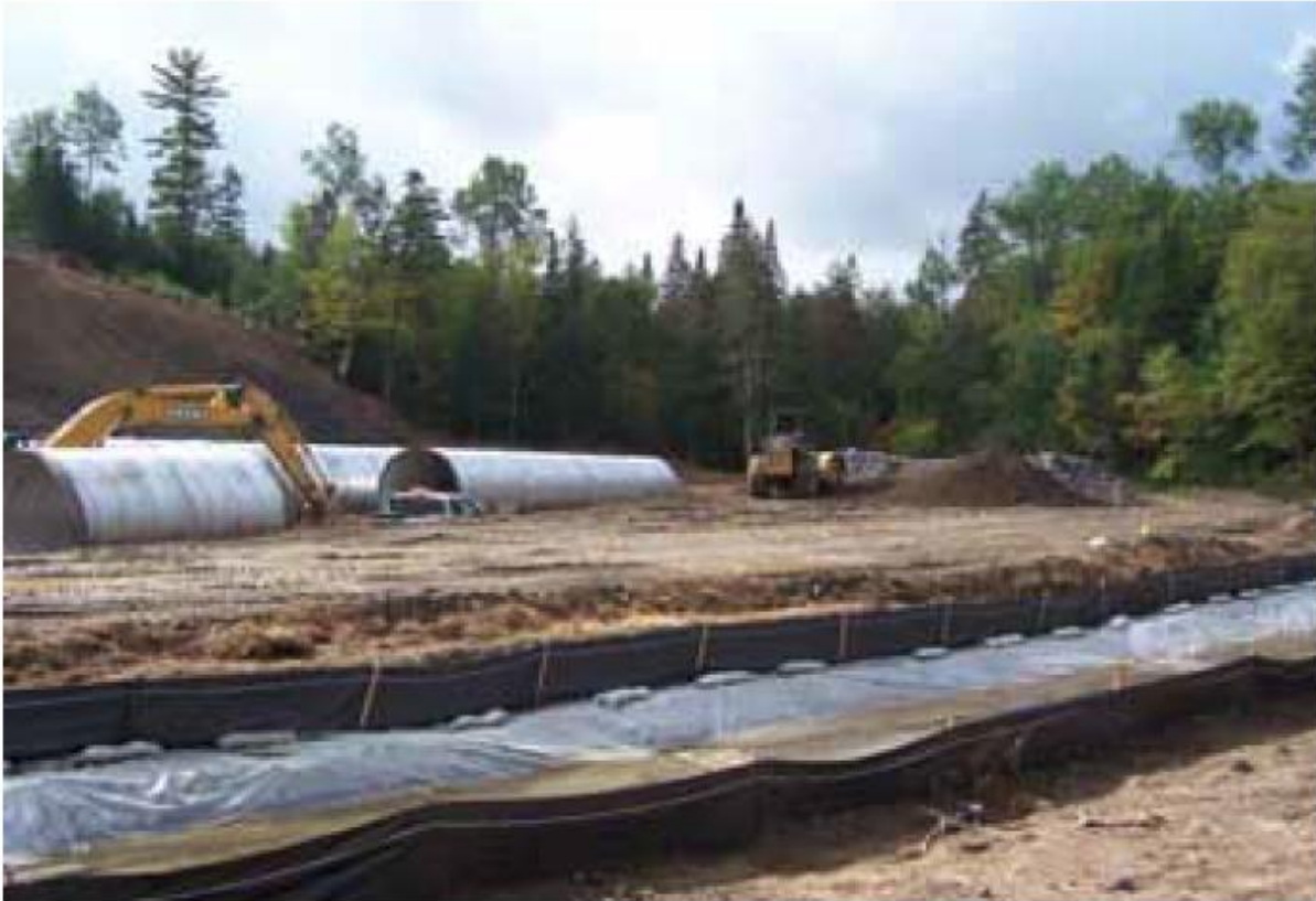
A temporary plastic-lined diversion channel.
