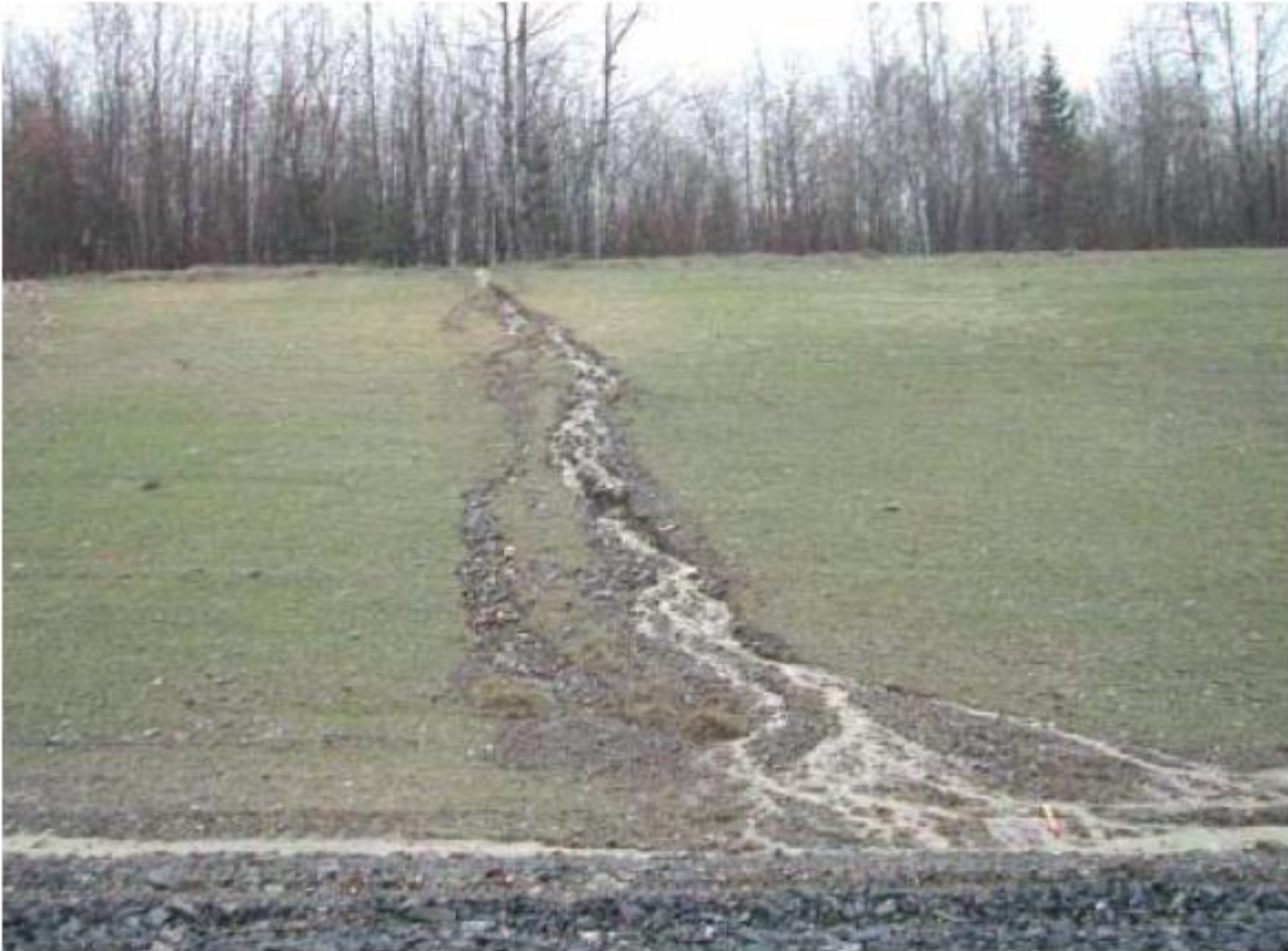
This slope requires a flume (slope drain) to carry flow from the top of the slope to the ditch.
