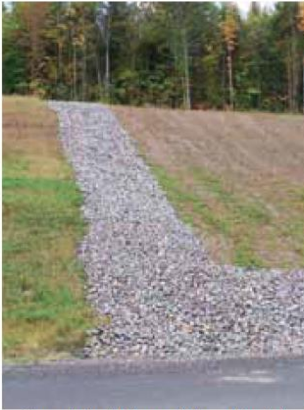
Completed Flume (Slope Drain)
