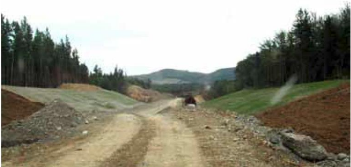
Areas stabilized as work progresses - Good Work Progression
