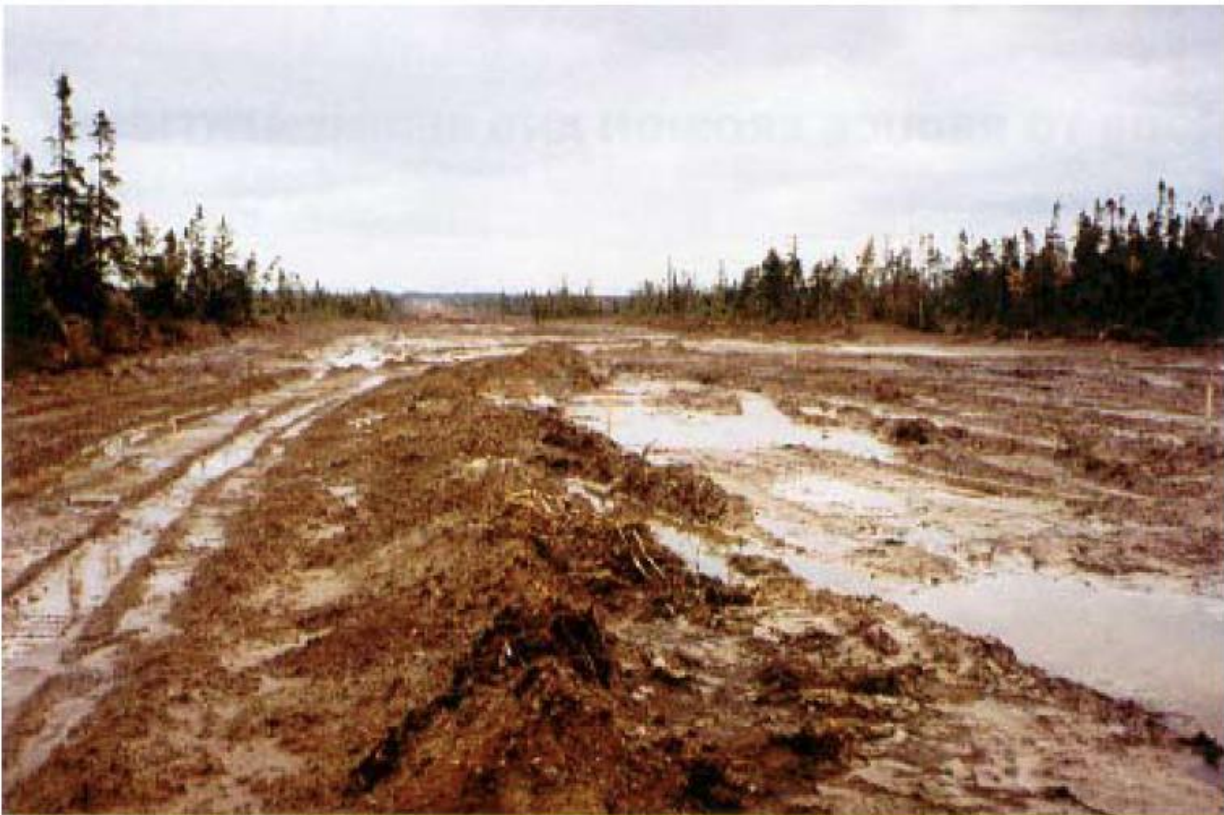
Area stripped of all vegetation – Poor Work Progression
