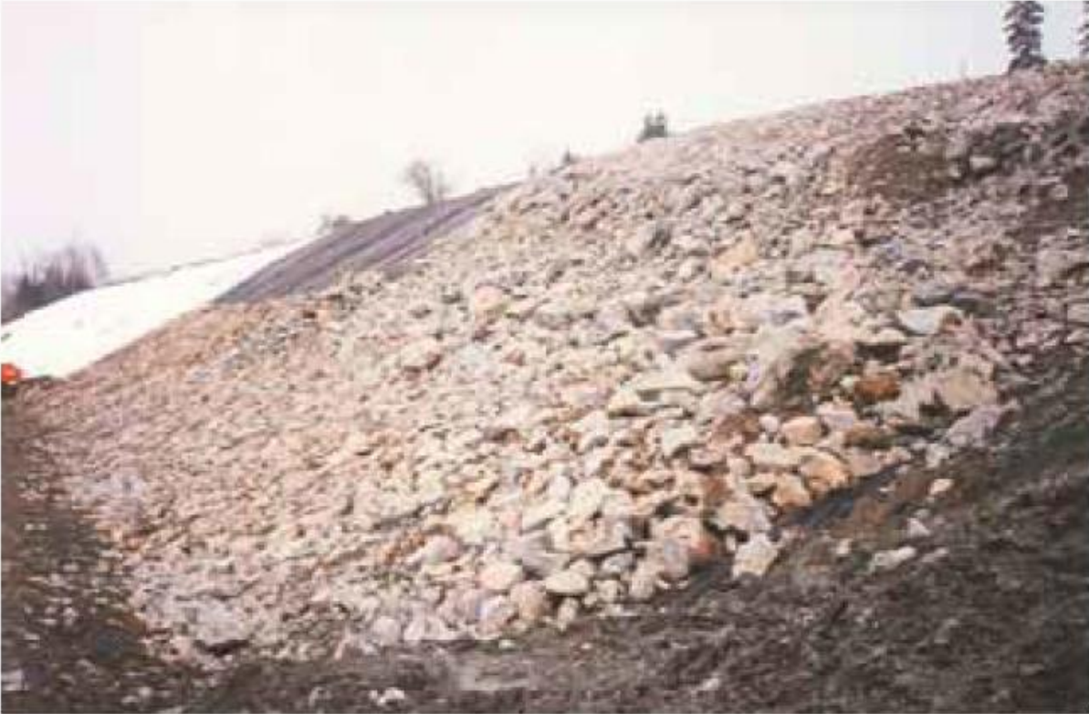
Placement of riprap on backslope.
