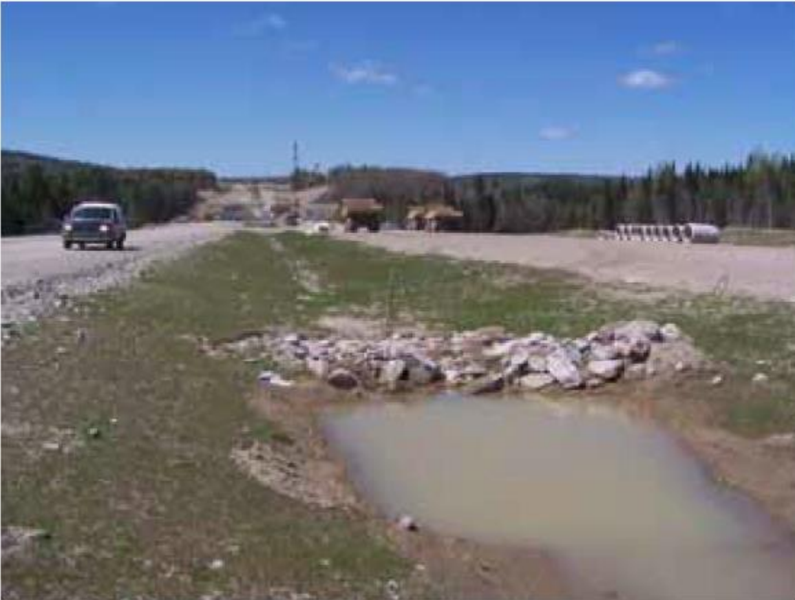
Completed Type B Erosion Control Structure
