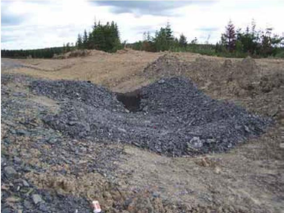
Completed Type A Erosion Control Structure
