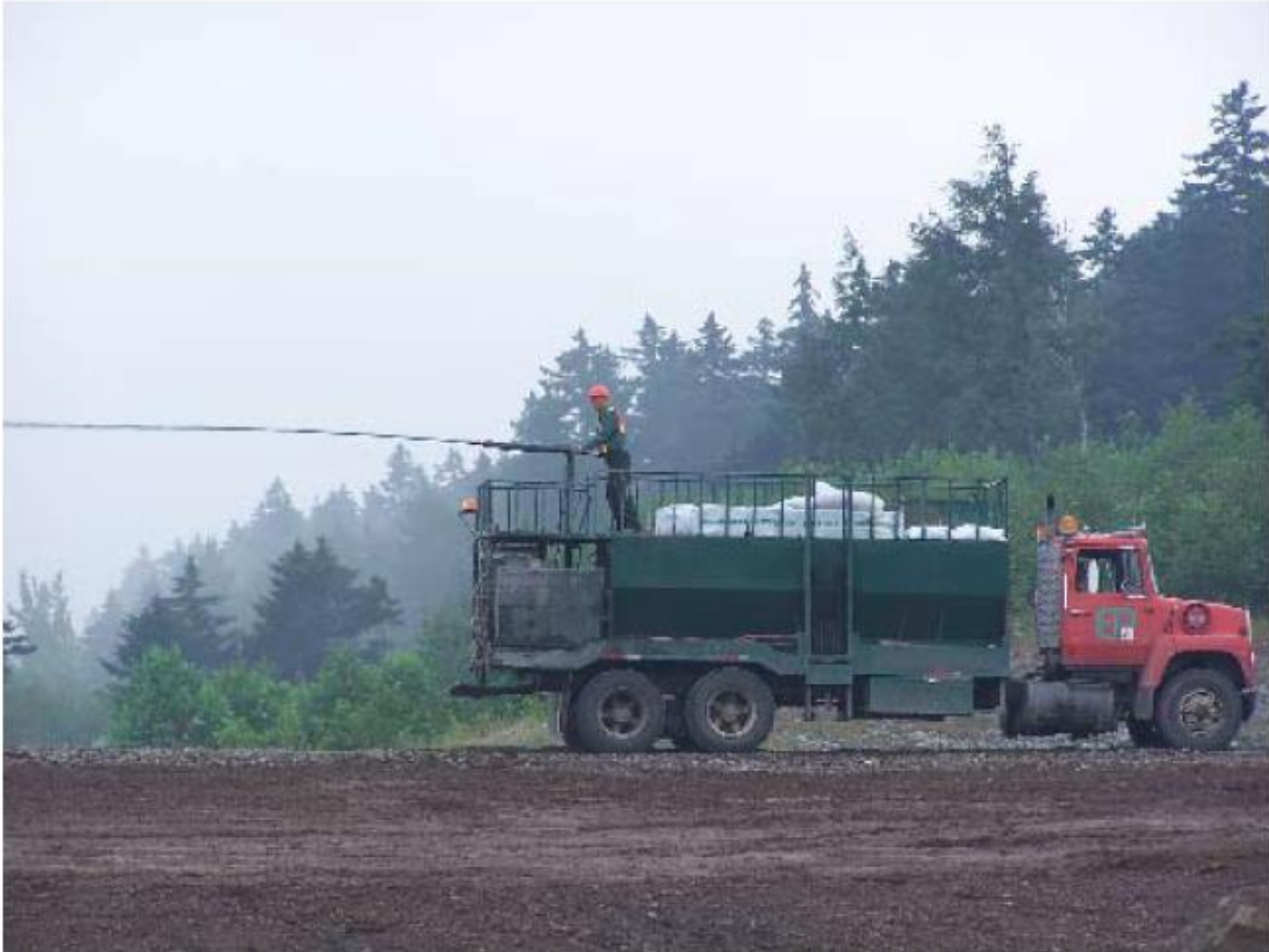
Hydroseeding – Application by mechanical means
