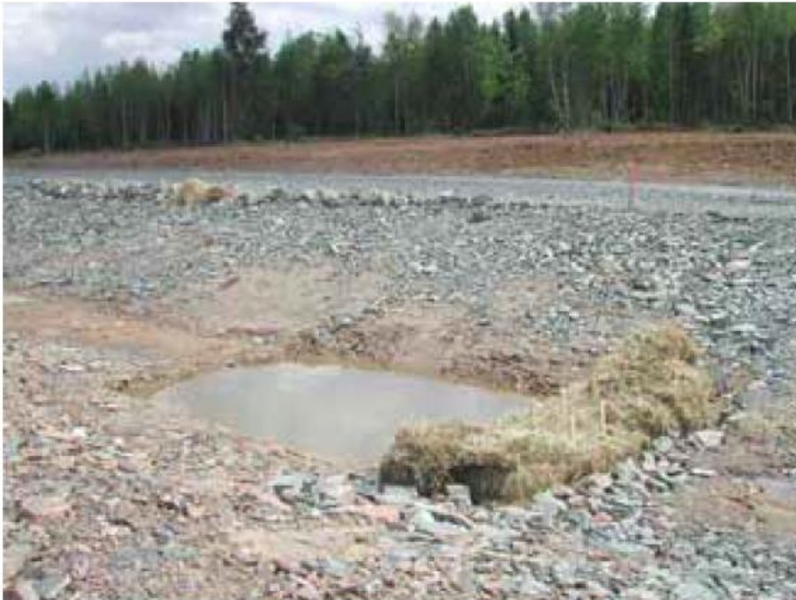
Completed Type D Erosion Control Structure
