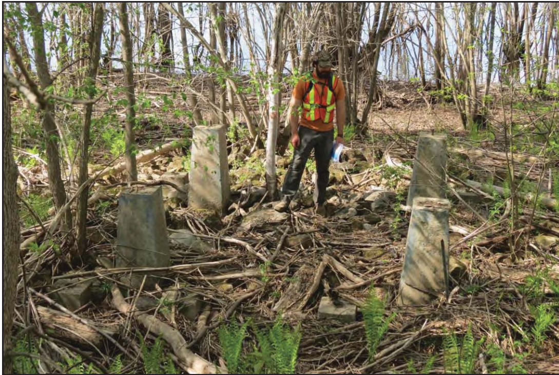
PLATE 3: Concrete pilings within floodplain of Saint John River; facing north; May 29, 2014.
